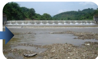
Weir (after construction)
