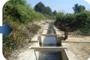
Main Canal (after construction)
